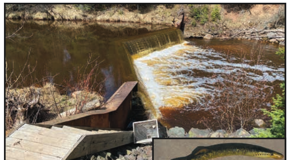
While sea lamprey are skilled (suction mouth) climbers but only modest jumpers, barrier dams on northwest Wisconsin’s Middle River and other Lake Superior tributaries are effective in preventing the exotic predators from reaching upstream spawning grounds. Lampreys living in Great Lakes ecosystems are native to the Atlantic Ocean where fish species—both large in size and population—have evolved together. In the Great Lakes, sea lampreys have on outsized impact on the health of native fisheries. GLIFWC and its federal, state, and tribal partners work cooperatively to control sea lamprey abundance. INSET: Adult sea lamprey in Lake Superior grow up to around 16-24” long. (CO Rasmussen photos)
