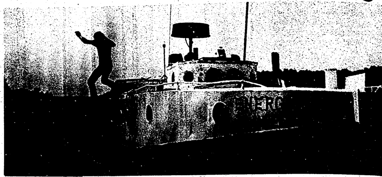
The Energy being made ready to leave.
