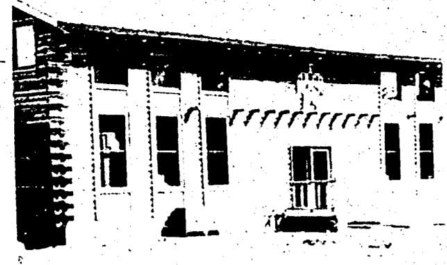
The Log Construction Training building stands as a powerful example of the skills of students and instructors.
