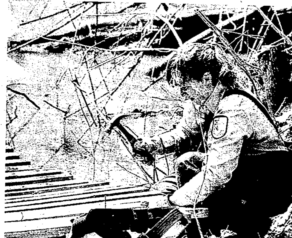
Kasha Mullet, U.S. Fish & Wildlife Service Sea Lamprey Control Program, Marquette, Michigan assists in set up for sea lamprey trapping. Flooding conditions on the Bad River made bridge building necessary in order to access areas where traps were to be set. (Photo by Lynn Plucinski)
