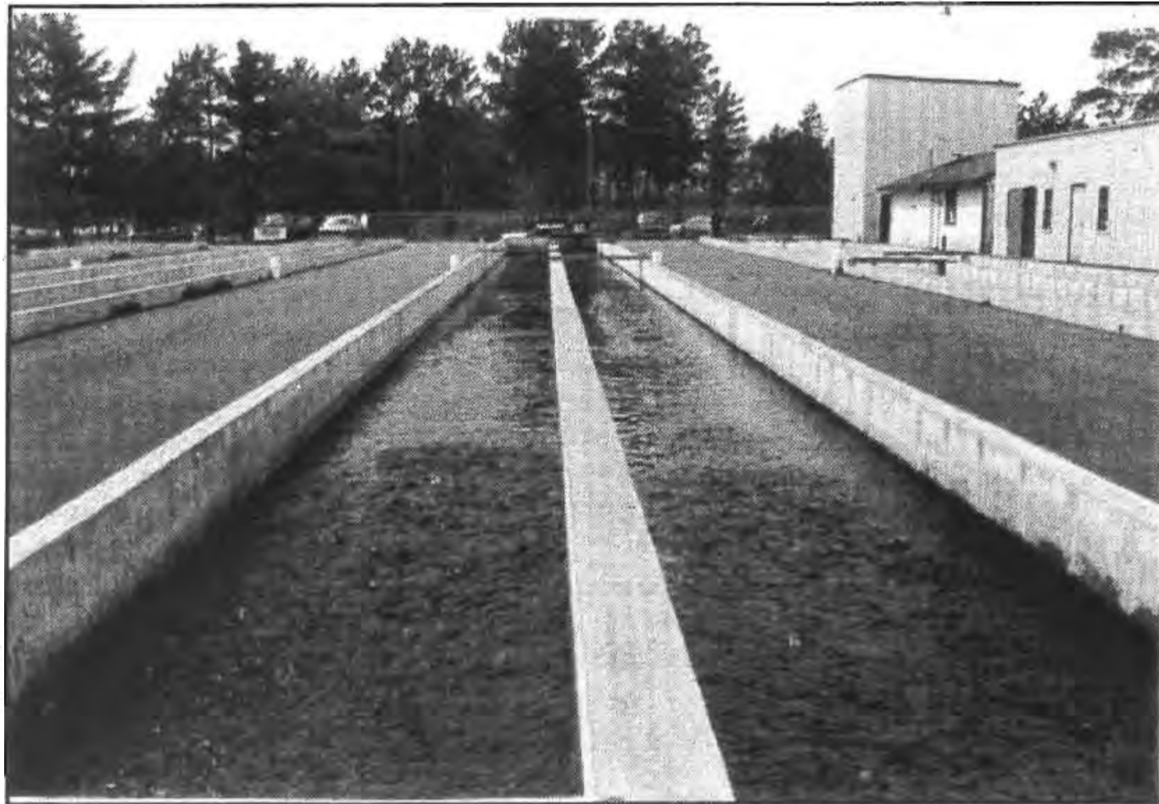
The extensive raceways at the Lac du Flambeau Tribal Hatchery allow the facility both to maintain brood stock and rear extensive numbers of fry to fingerling size. (Photo by Amoose)
