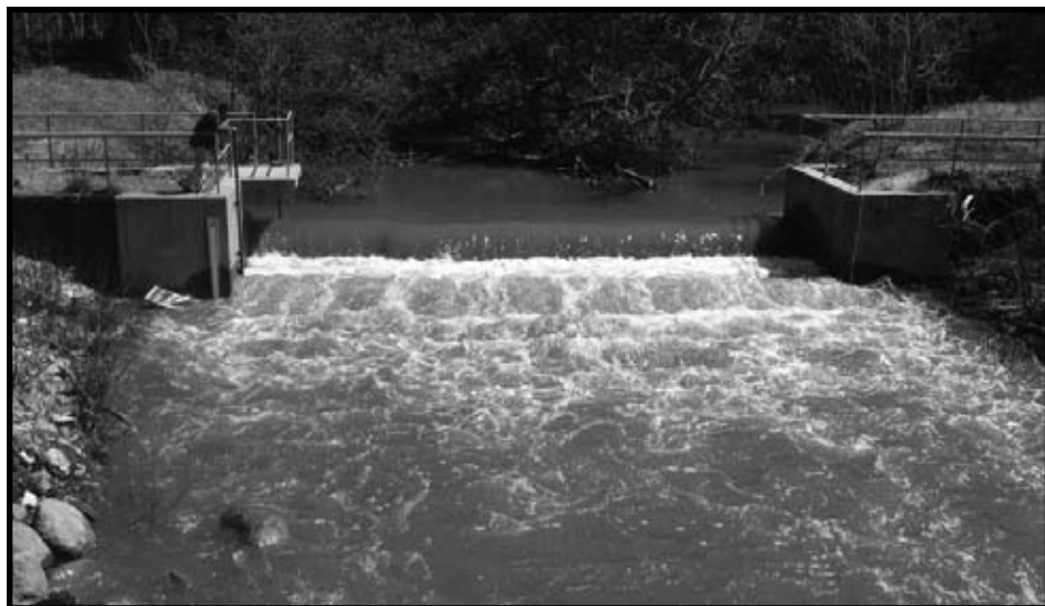
The Misery River in Michigan is swollen by spring rains and snowmelt, but the lamprey traps are fishing. The first day's catch was a couple dozen white suckers and a few trout. Soon the traps will be full of adult lampreys that will be swimming upstream to spawning grounds which are blocked by this low-head barrier dam. The dam blocks the migration of non-jumping fish like the sea lampreys. Many of these structures exist around the Great Lakes, built for the sole purpose of stopping sea lampreys from getting access to spawning grounds. (Photo by Bill Mattes.)
