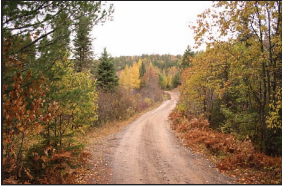
The current sand and gravel road just south of the Dead River crossing. North of here the road progressively narrows and eventually becomes impassable to motorized vehicles. (Photo by Steve Garske.)
