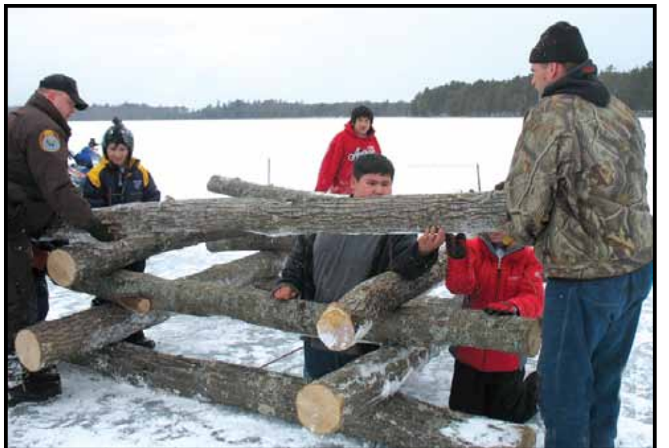
GLIFWC conservation officers teamed up with students and staff from Lac du Flambeau School to construct two fish cribs on the ice at Wild Rice Lake. Several weeks after the March 27 event, the cribs sunk to the lake bottom after ice-out, improving habitat for fish and other aquatic species. (Photo submitted.)
