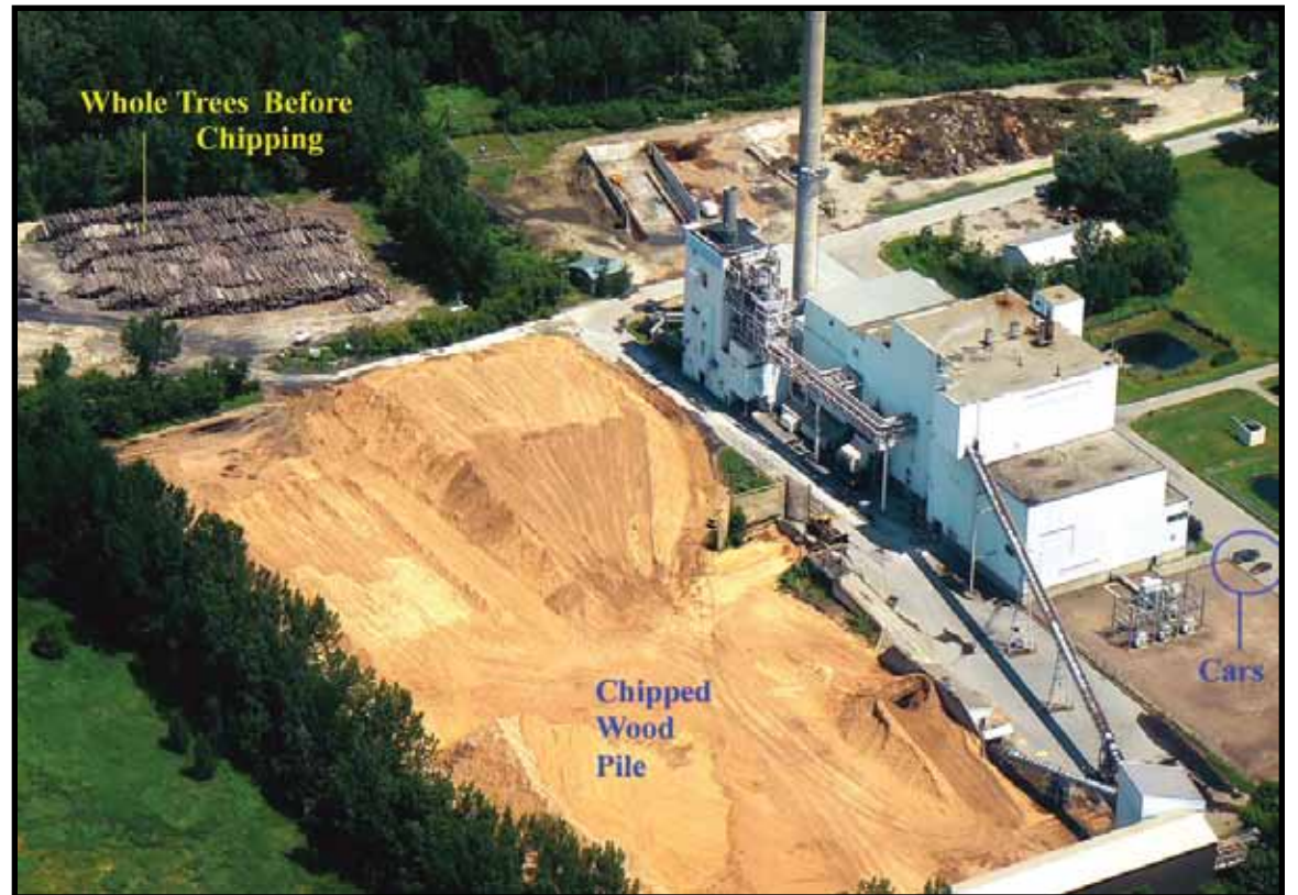
The 50 MW McNeil wood gasification plant in Vermont. Note pile of whole logs, which are chipped for fuel. (Photo by Chris Matera, Massachusetts Forest Watch)
