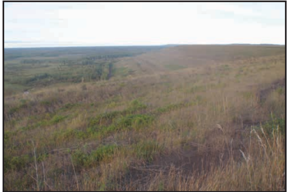
North face of the Ling Temco Vought (LTV) tailings basin. PolyMet would deposit its tailings on top of this existing basin. Thousands of gallons per minute of high sulfate water is currently seeping out of this facility and into the surrounding wetlands and streams. If PolyMet tailings are deposited on the top, water from those tailings would seep out as well. A seepage capture system is proposed to try to limit that discharge.
