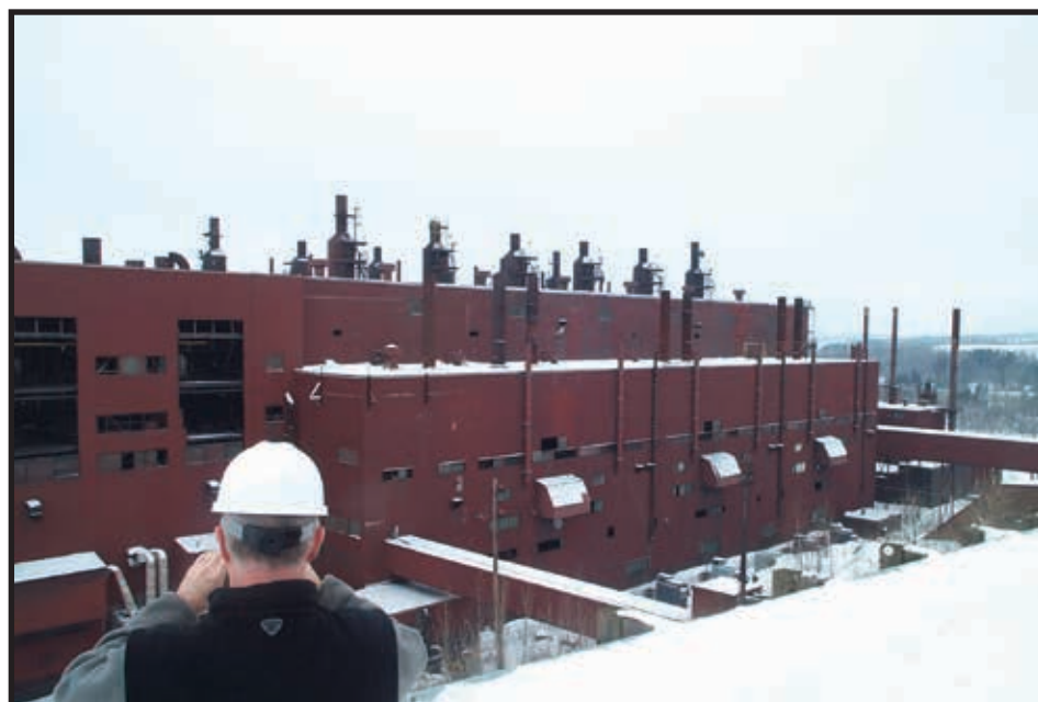
A portion of the processing facility at the PolyMet plant site. The old taconite processing facility would be converted to process copper ore.
