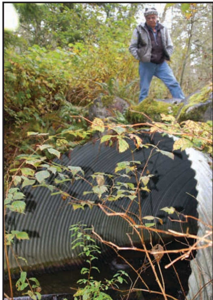
The late Northwest Indian Fisheries Commission (NWIFC) Executive Director Billy Frank Jr. examines a culvert in the upper Nooksack River watershed in Washington State in 2008. NWIFC member tribes successfully argued that the State has a duty to protect treaty resources—in this case salmon habitat in the territory ceded by 22 tribes in Washington. For decades, poorly installed culverts have blocked the passage of salmon from the ocean to inland waterways. (photo courtesy Tony Meyer/NWIFC)
