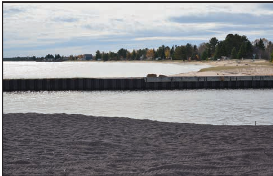
A view looking south shows the stamp sands deposited in the foreground, the Grand Traverse Harbor in the center and the natural sand beaches and homes south of the harbor in the background. (Michigan DNR photo)
