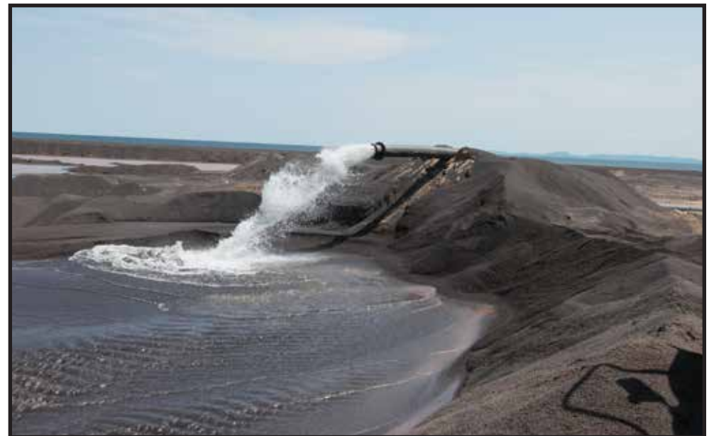
A watery slurry of mining waste and other materials dredged from Grand Traverse Harbor flows into a containment basin near the main body of stamp sands. (E. Chiriboga photo)
