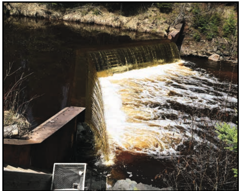
Barrier dams on Great Lakes tributaries prevent adult lampreys from migrating upstream to suitable spawning grounds. This dam is located on Wisconsin's Middle River along the Lake Superior south shore. (CO Rasmussen photo)
