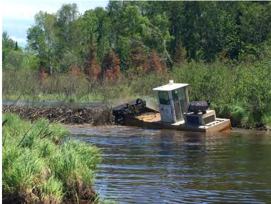
Bois Forte Operators use the Swamp Devil to remove beaver dams for water level management
