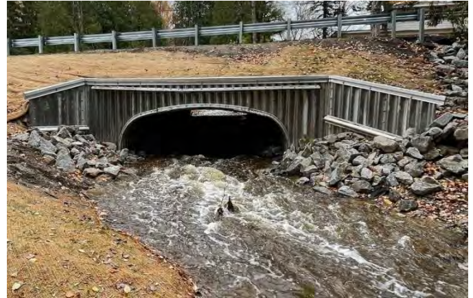
A restored culvert along Tannery Creek.
