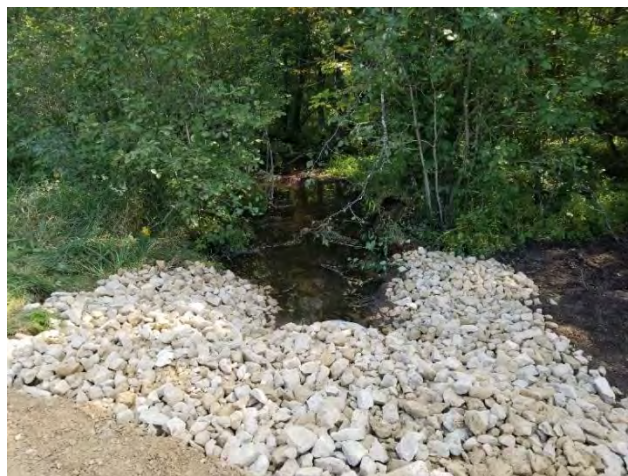
Complete road stream crossing.
