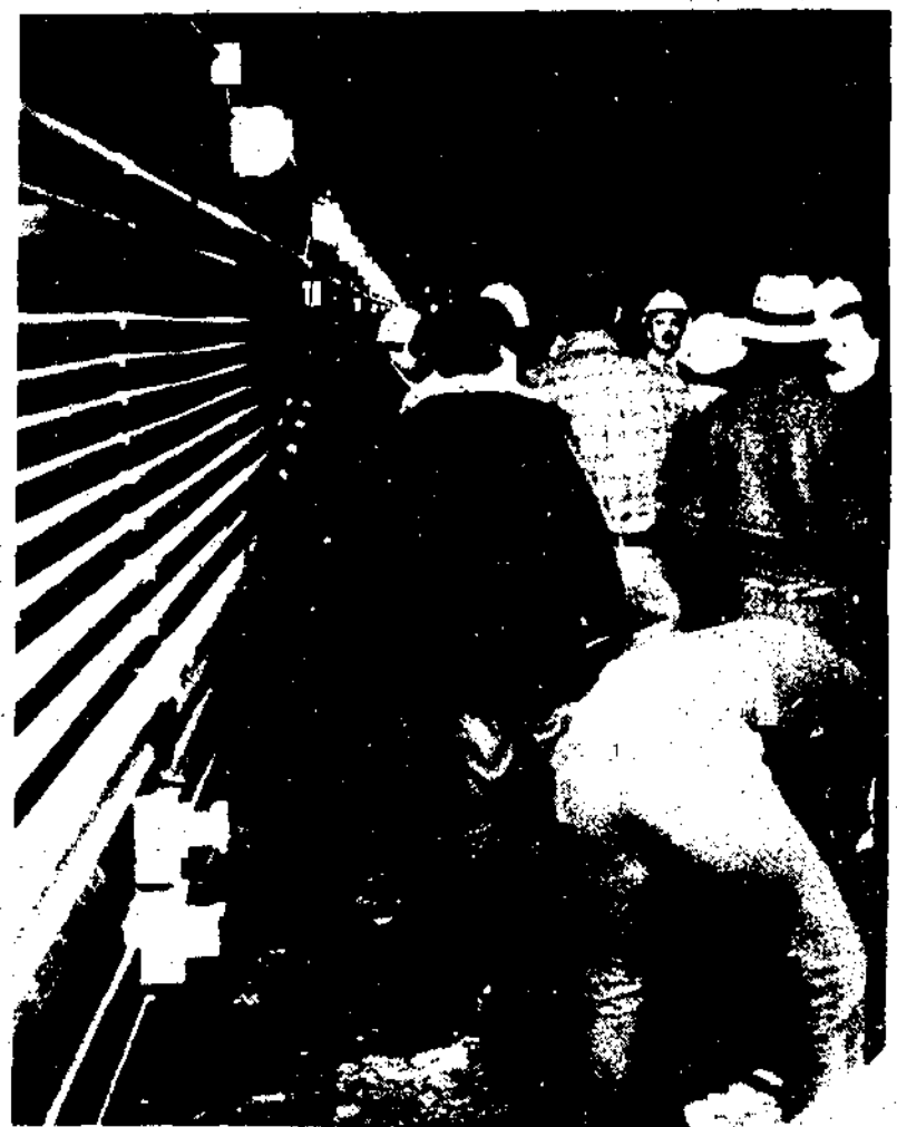
In the tunnel leading into a mountain where the Hanford site is doing tests on heat & compression on the salt rock - trying to prove this is the best place for a repository.
