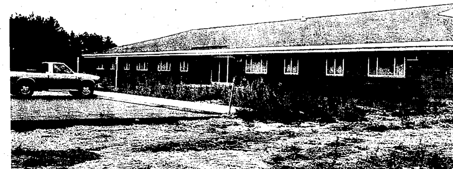
Just completed apartment building for singles at Mole Lake.
