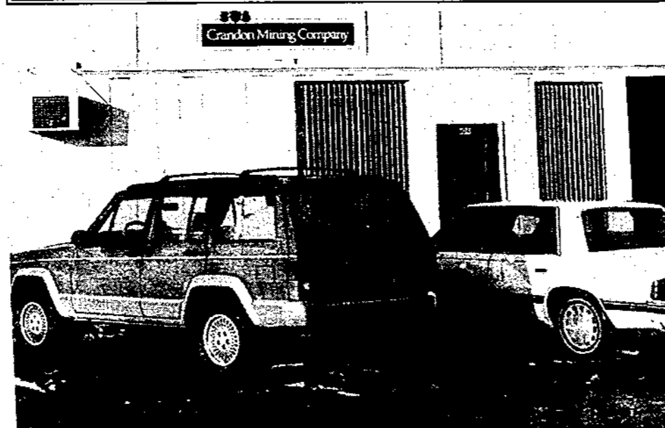
Inauspicious along one of Crandon's main streets is the main office for the Crandon Mining project, which recently announced filing for a mining permit with the WDNR. While the office does little to attract attention, the Mole Lake band of Chippewa find the mining proposal stemming from the place threatening to the resources and the continued well-being of their reservation and way of life. (Photo by Amoose)
