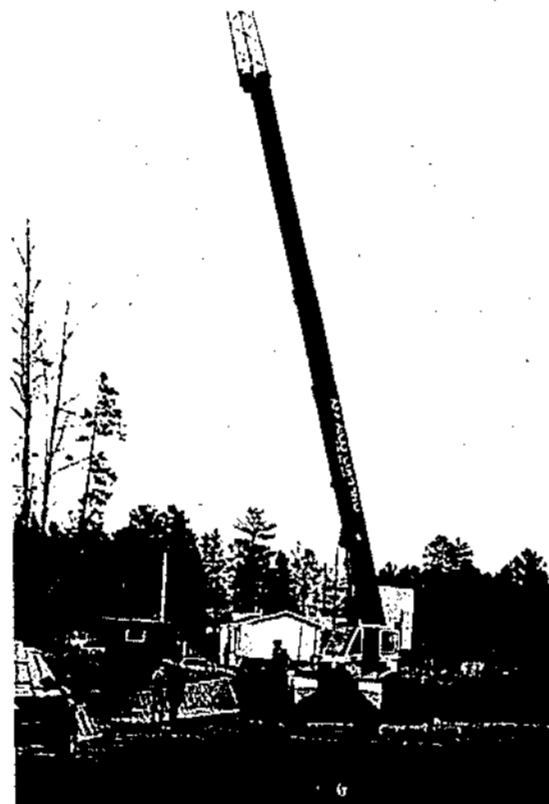
To better utilize GLIFWC's existing radio system a radio tower was erected in back of the new Bad River/ GLIFWC administration building in Odanah. (Photo by Sue Erickson)
