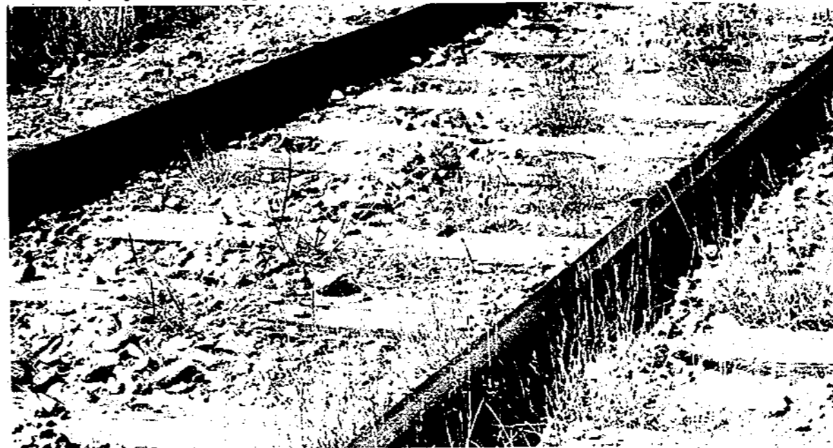
The safety of the tracks used by Wisconsin Central railway to transport sulfuric acid to the White Pine Mine in Michigan is being seriously questioned. (Photo by Amoose)
