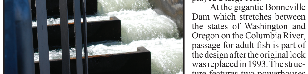
A Bonneville Dam fish ladder allows passage for salmon up the Columbia River to spawn. Accommodations for the fish have resulted in stronger runs being seen upriver. (SE)
