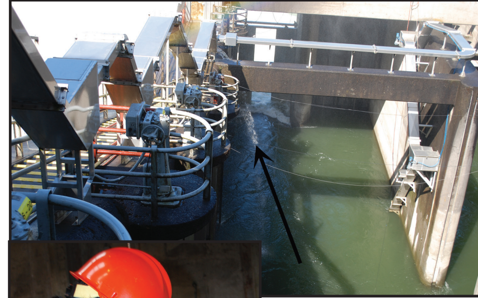
Although Bonneville Dam is designed to allow fish passage through a system of locks and ladders, Pacific lamprey were still having difficulty negotiating through the dam on their way up river to spawn. Today, the lamprey swim up a gushing stream of water within the dam in order to migrate through the dam site. It seems an impossible feat, but the lamprey swim straight up a downspout of water. (SE)
