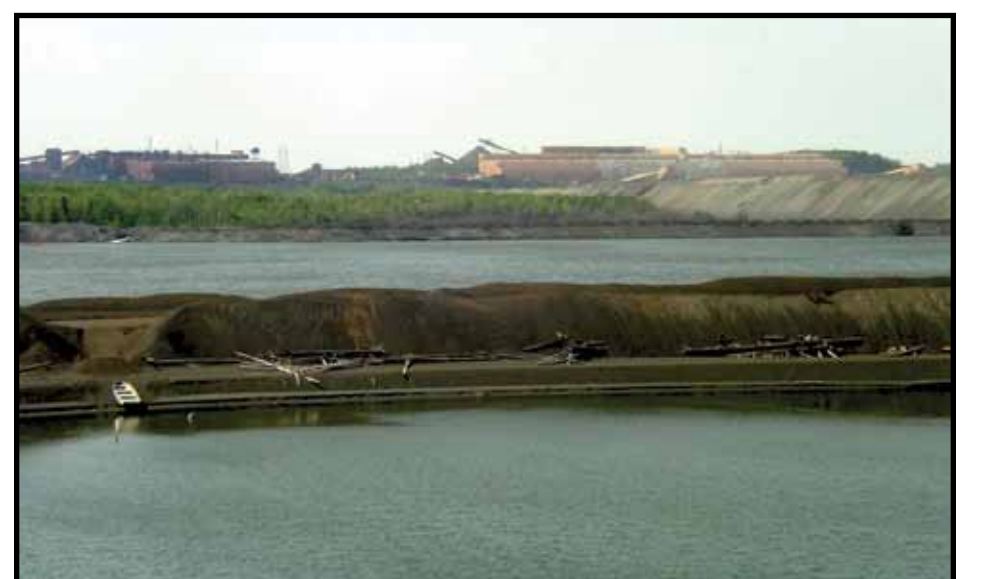
Tailings ponds and taconite processing facilities at Minntac, Minnesota.
