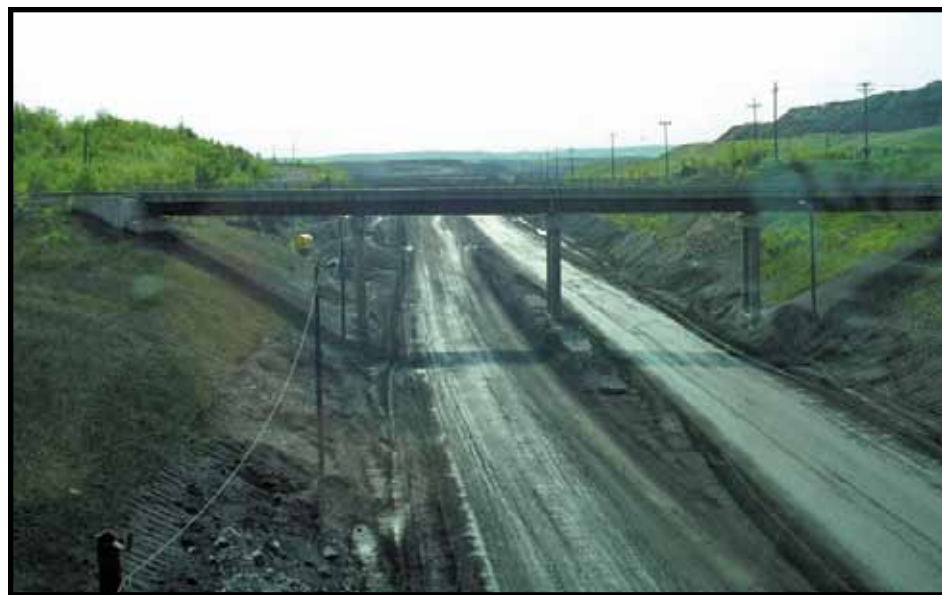
Haul road at taconite mine in Minnesota.
