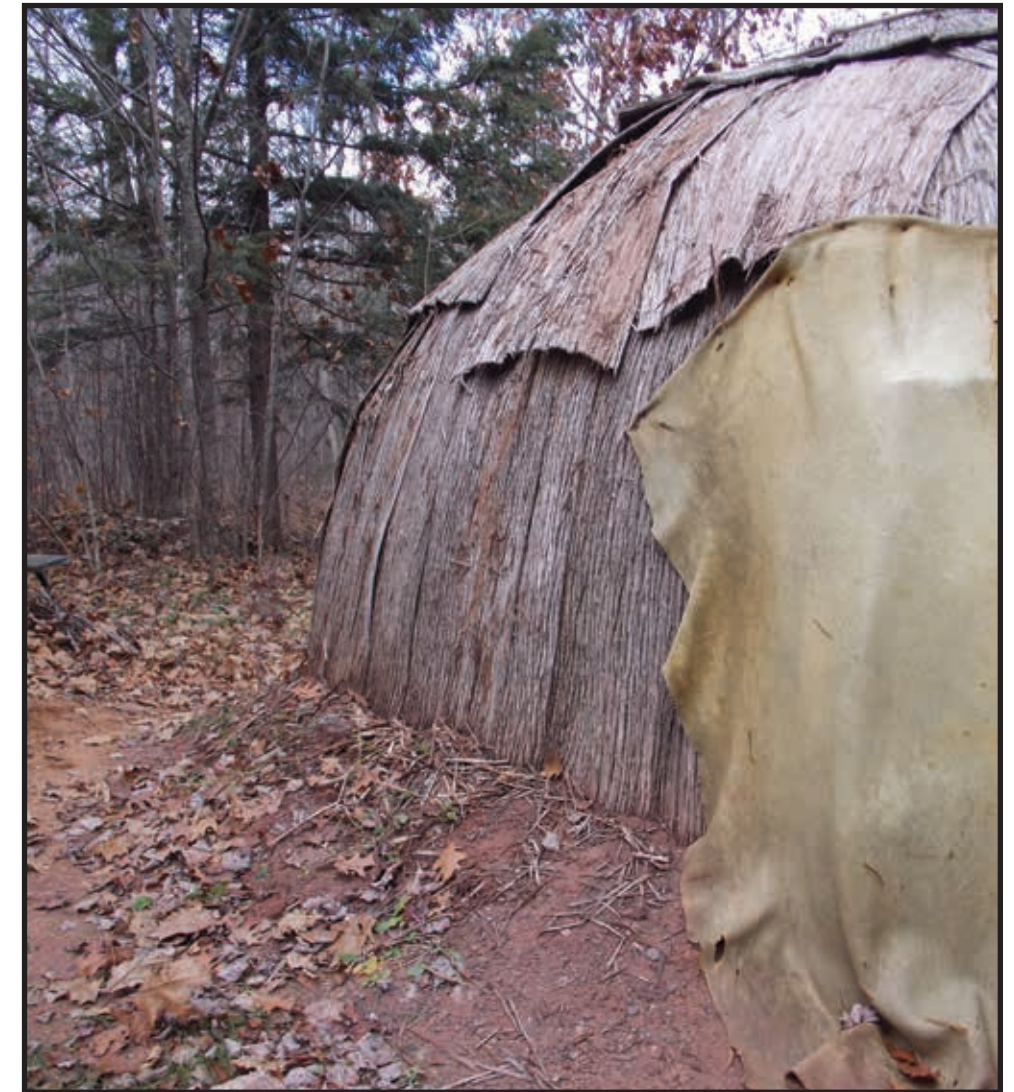
Clay is built up at the base as a moisture seal.
