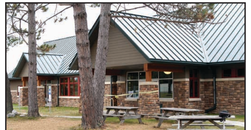
Through upgrades and new construction, the Lac du Flambeau Band is increasing energy efficiency in tribal buildings on its northern Wisconsin reserve. The natural resources building was LEED-certified in 2012. Leadership in Energy and Environmental Design, or LEED, is the most widely used green building rating system in the world. (CO Rasmussen photo)
