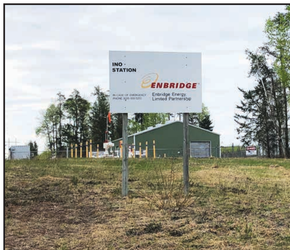
Enbridge's Ino Pump Station is located in the Chequamegon-Nicolet National Forest. (Charlie Otto Rasmussen photo)
