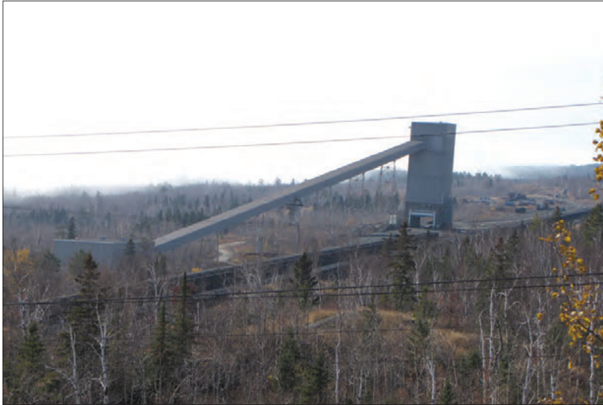
Headframe at the Northshore mine in Silver Bay, which has been operating since 1956.
