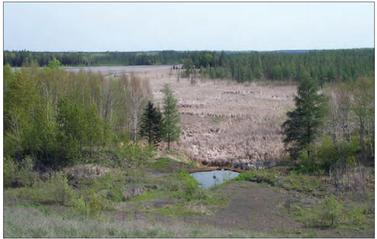
Water seeping out of the Minntac tailings basin and moving toward the Sandy Lakes in Minnesota.
