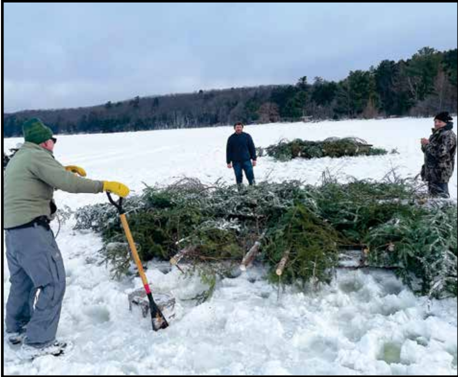
GLIFWC fishery staff collaborated with the Town of Plum Lake Lakes Committee, Lake Laura residents, Vilas County, and Wisconsin Department of Natural Resources to construct and site fir tree bundles on January 31. A series of three large balsam bundles located at two sites on Lake Laura will sink at ice-out and rest at the lake bottom. Popularly known in the fish conservation community as “fish sticks,” the structures provide habitat for perch and other forage fish. (M. Luehring photo)
