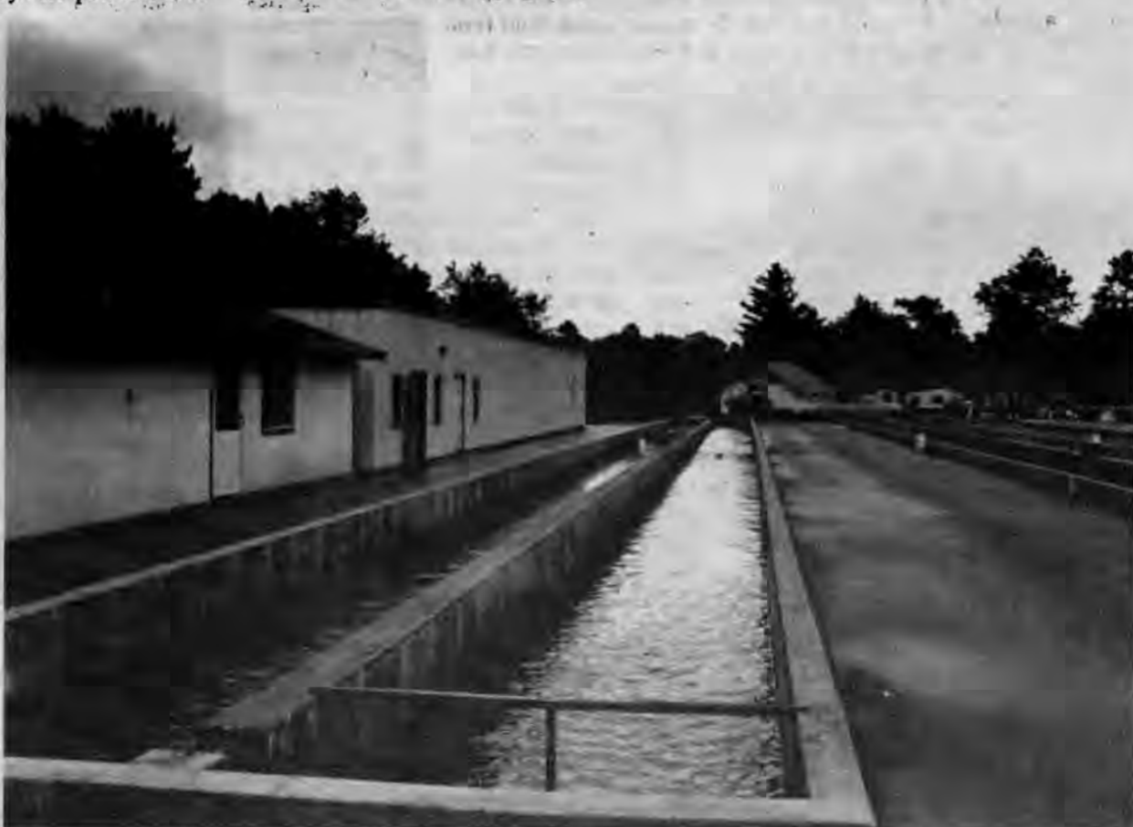
Lac du Flambeau's fish culture program involves raising many species of native fish to the area in the hatchery facilities, including a 315-jar hatchery, Heath incubators, 11 start tank raceways, and ten 200-foot concrete raceways and 21 fish culture ponds. (Photo by Amoose)
