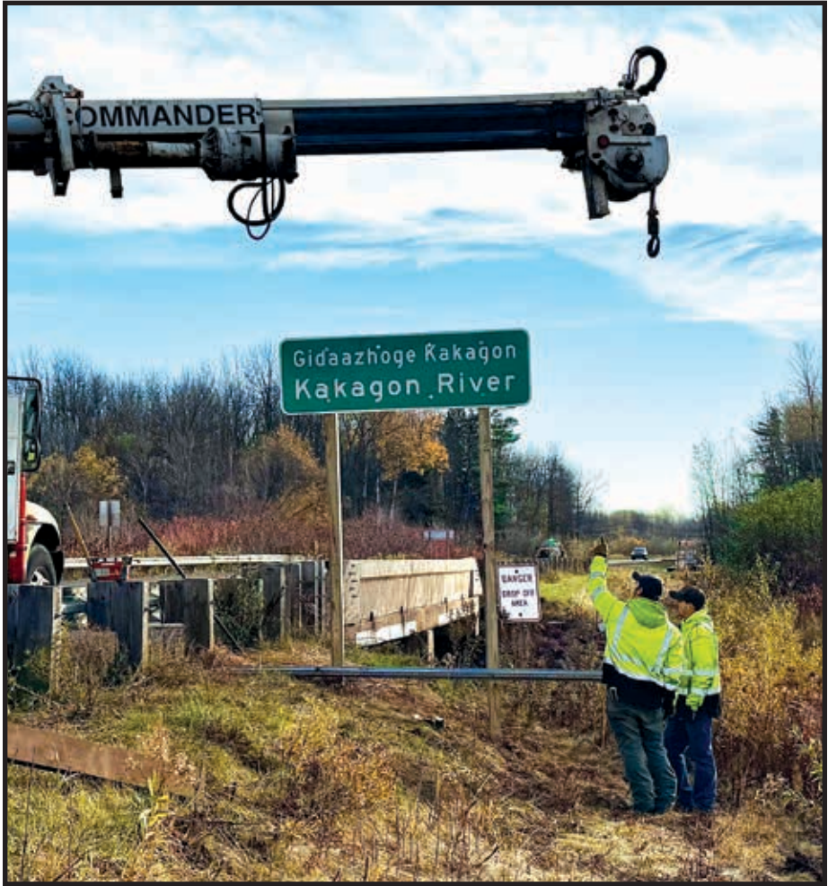
A crew from the Ashland County Highway Department installed dual language signs October 28 on US Highway 2, alerting motorists they were crossing the Kakagon River. Bad River Tribes’s Ben Connors monitored the installation to ensure proper handling of any potential cultural items uncovered in the work. (CO Rasmussen photo)
